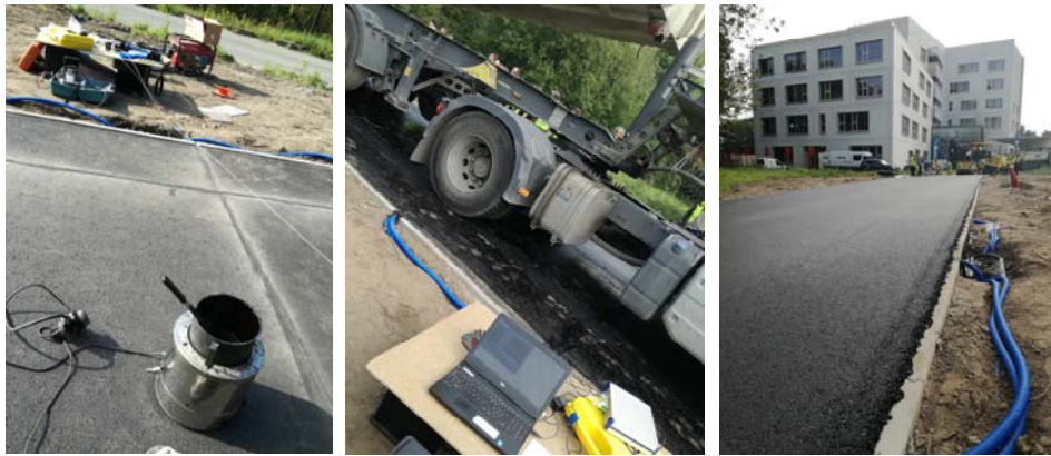
Figure 6. Installation of FBGs in two asphalt base layers (second approach).
