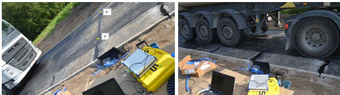
Figure 8. Monitoring of FBGs during the second day during the construction of the second base layer of the CyPaTs bicycle path.
