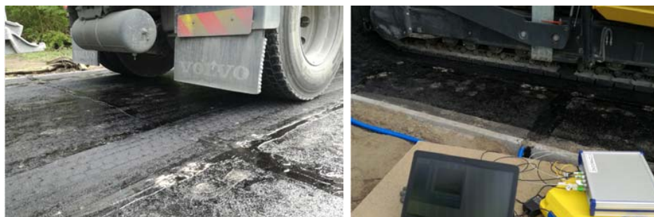
Figure 10. Monitoring of FBGs on the third day during the construction of top layer of the CyPaTs bicycle path at a temperature of 24 °C on the surface of the second base layer AC-10.
