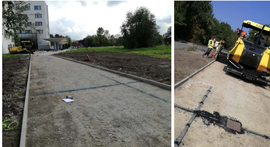
Figure 5. Installation of FBGs in the base asphalt layer directly on the base (first approach).
